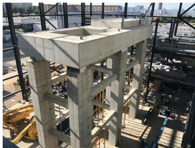
The completed turbine platform. Source: PORR/Fabian Hemauer
