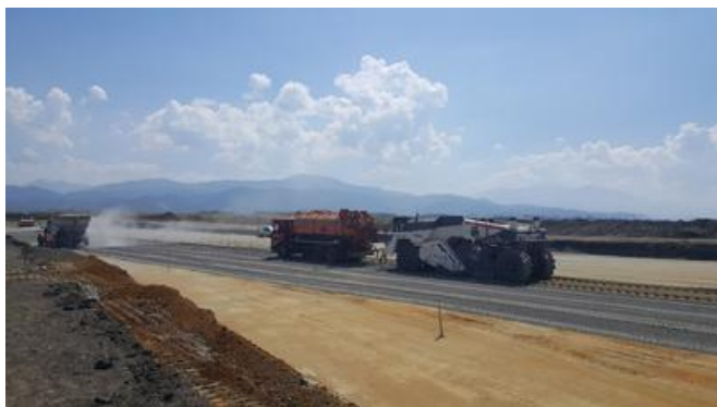
A 25cm thick stabilised ballast layer was laid on top of the lower ballast layer for the taxiway and apron. Source: PORR Construct
