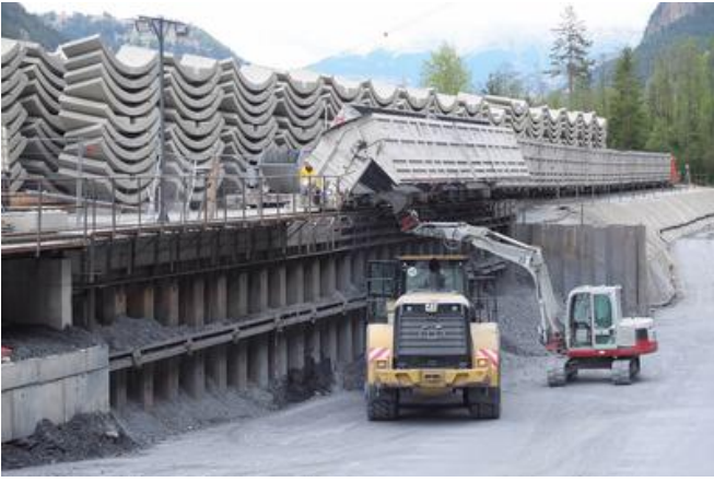
The GKI Maria Stein consortium took over the existing construction site from the previous contractor. Various restructures were necessary to improve efficiency – for example, the system for unloading spoil from the service carriages was completely reorganised. Source: GKI Maria Stein consortium
