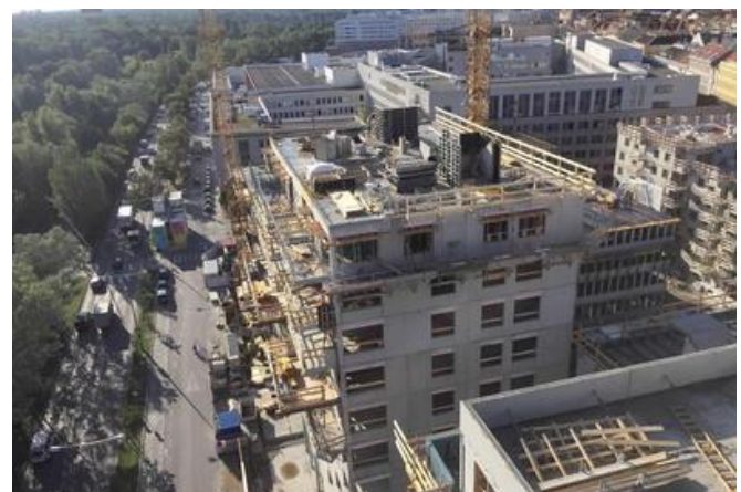
The overhanging balconies in the three top storeys presented a major challenge during the carcass construction. Source: PORR
