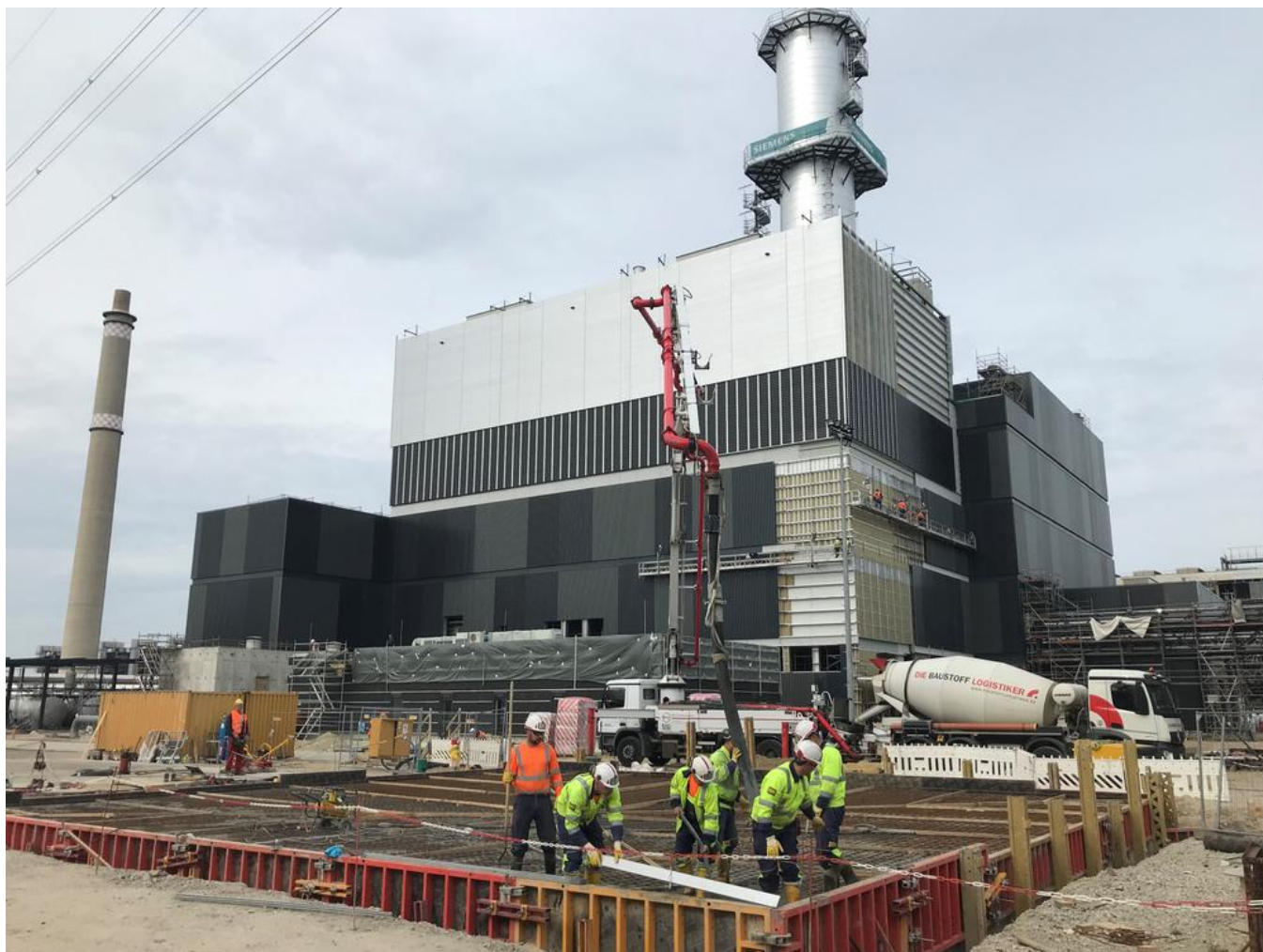
Concreting the outdoor storage area floor slab for the Marzahn combined heat and power station. Source: PORR/Fabian Hemauer
