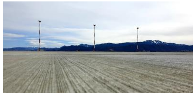
PORR built a high-mast lighting system at the edge of the platform. Source: PORR Construct
