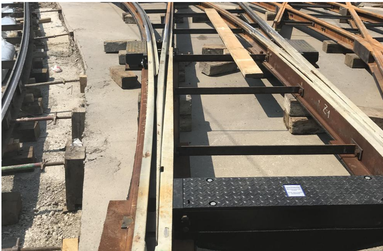
The grooved swivel plates for the intersection were pre-installed. Source: PORR AG
