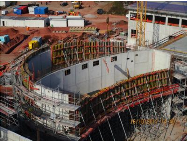
The stage tower has a curved reinforced concrete wall that was a significant challenge to build. Source: BBGS GmbH
