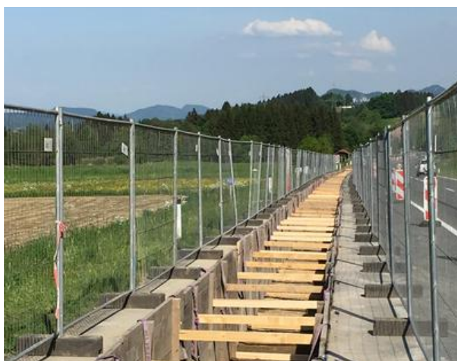
The district heating transport pipeline in Pöckau. Source: PORR
