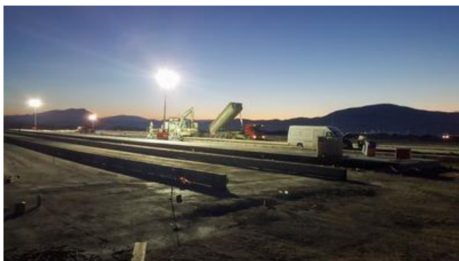
Solid steel girders were used as formwork for the concrete layer.
