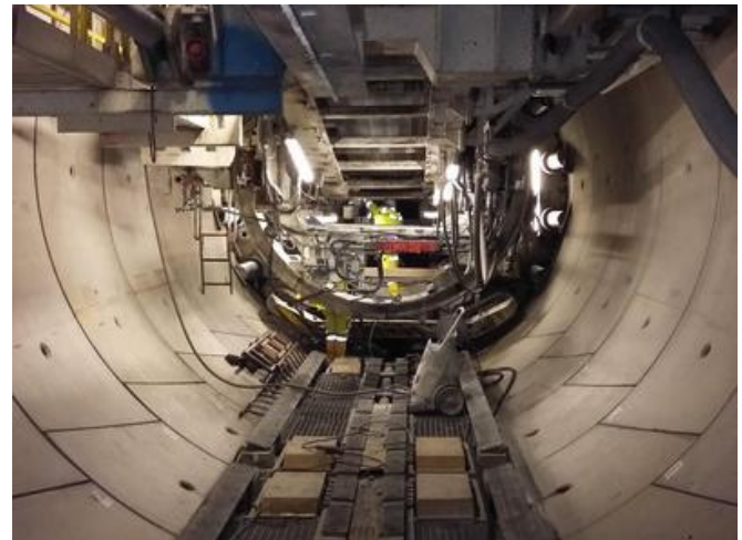
The two tunnel boring machines had to bore through almost 20km of grey Bündner schist. Source: GKI Maria Stein consortium
