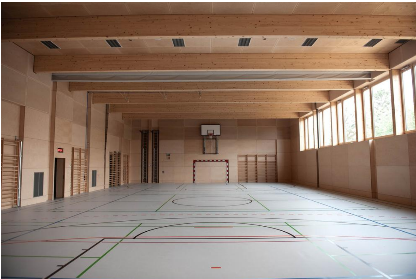
In total, 4,300m 2 of solid CLT ceilings and 3,100m 2 of solid CLT walls were installed. Source: Gerfried Tamerler/PORR
