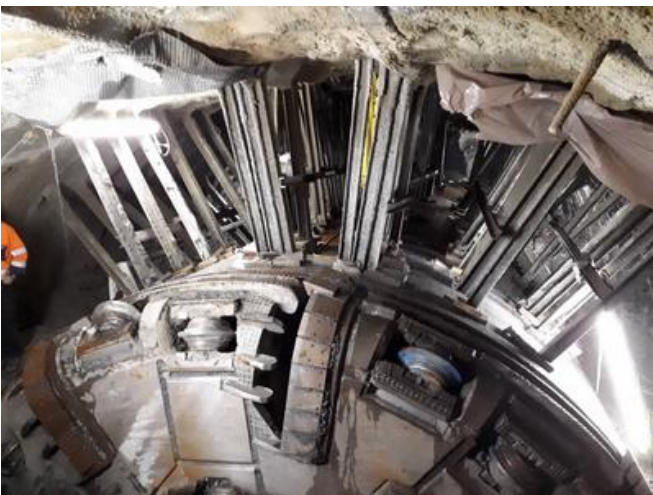
On several occasions, the trapped shield skin had to be released by raising the tunnel roof. Source: GKI Maria Stein consortium
