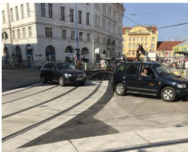
The road was usable very soon after the road surface concrete had been installed. Source: PORR AG
