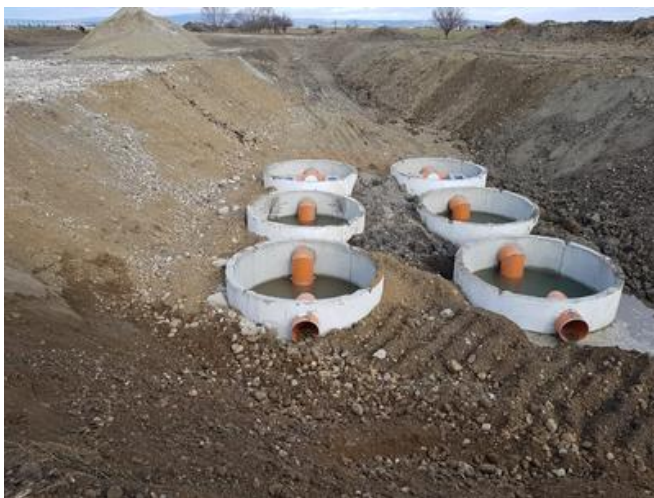
Water is cleaned in the two-stage oil separator system. Source: PORR Construct
