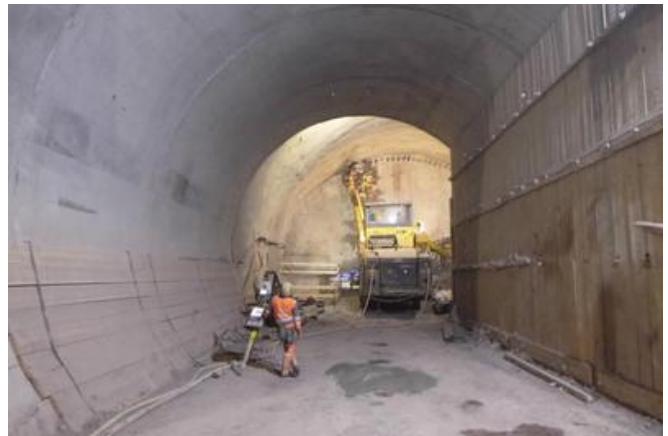
Excavation cross-sections of up to 200 m². Source: ATCOST21
