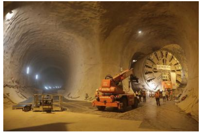
The rotation of the shield section through the turning cavern was particularly spectacular. Source: ATCOST21
