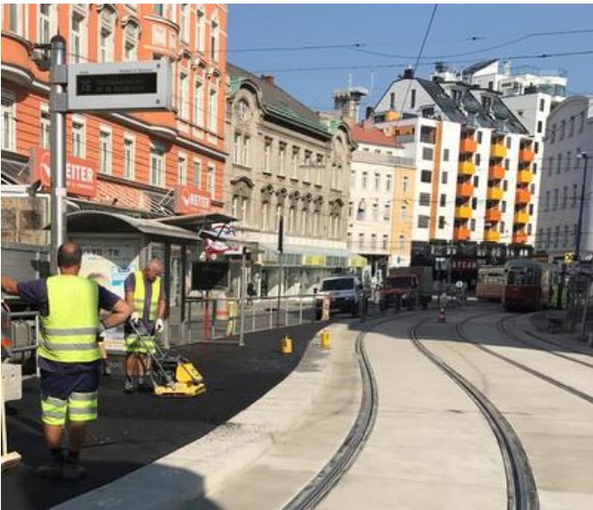
The final stage was to install asphalt between the guide wall element and the road at the tram stops. Source: PORR AG
