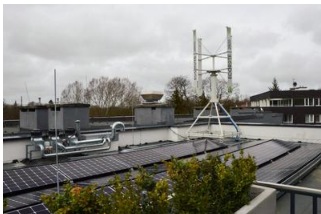
Several photovoltaic modules and a wind turbine on the roof provide clean electricity. Source: PORR
