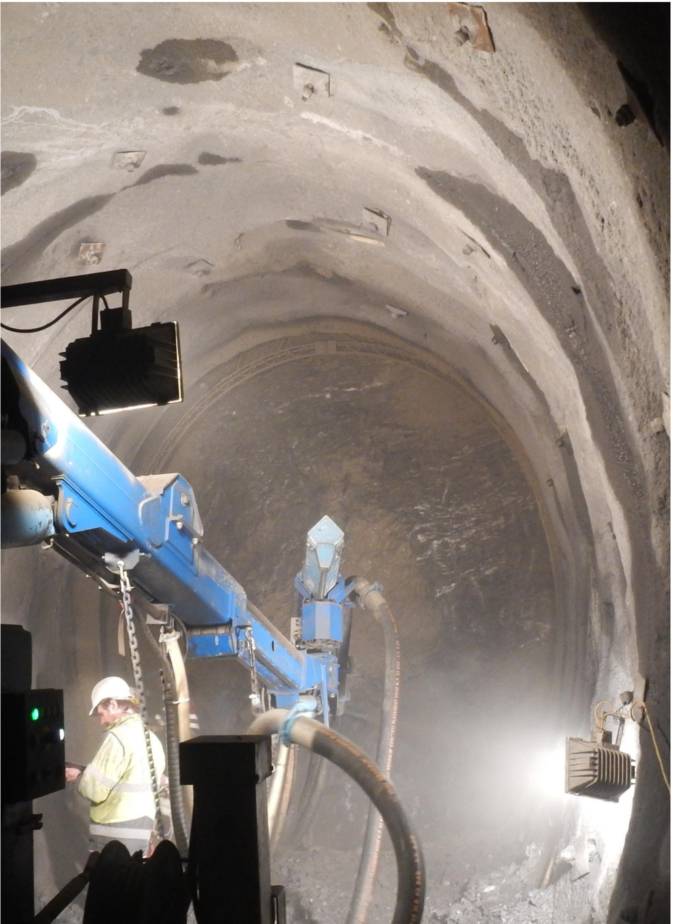
The tunnel boring work in the inclined shaft was given priority, so that the schedule could be met. Source: GKI PRB consortium
