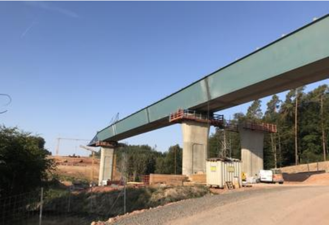
Six weeks of metalwork and welding preceded the successful launch. Source: PORR
