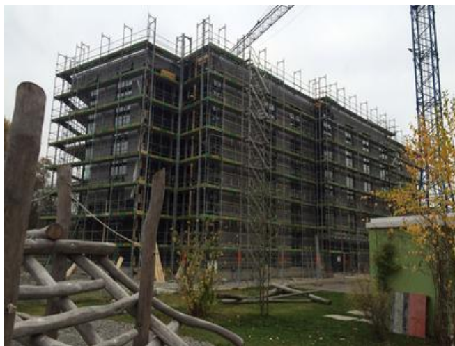
The carcass prior to installation of the ventilated facade. Source: PORR
