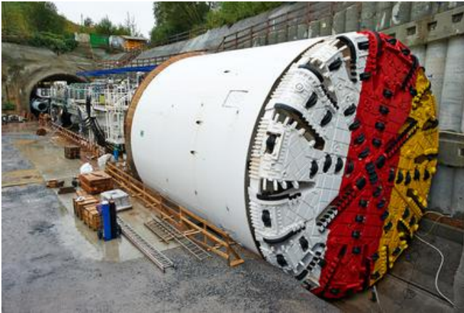
The “KORA” TBM was assembled in the Mitterpichling construction pit. The drill bears the Carinthian state colours. Source: Toni Rappersberger
