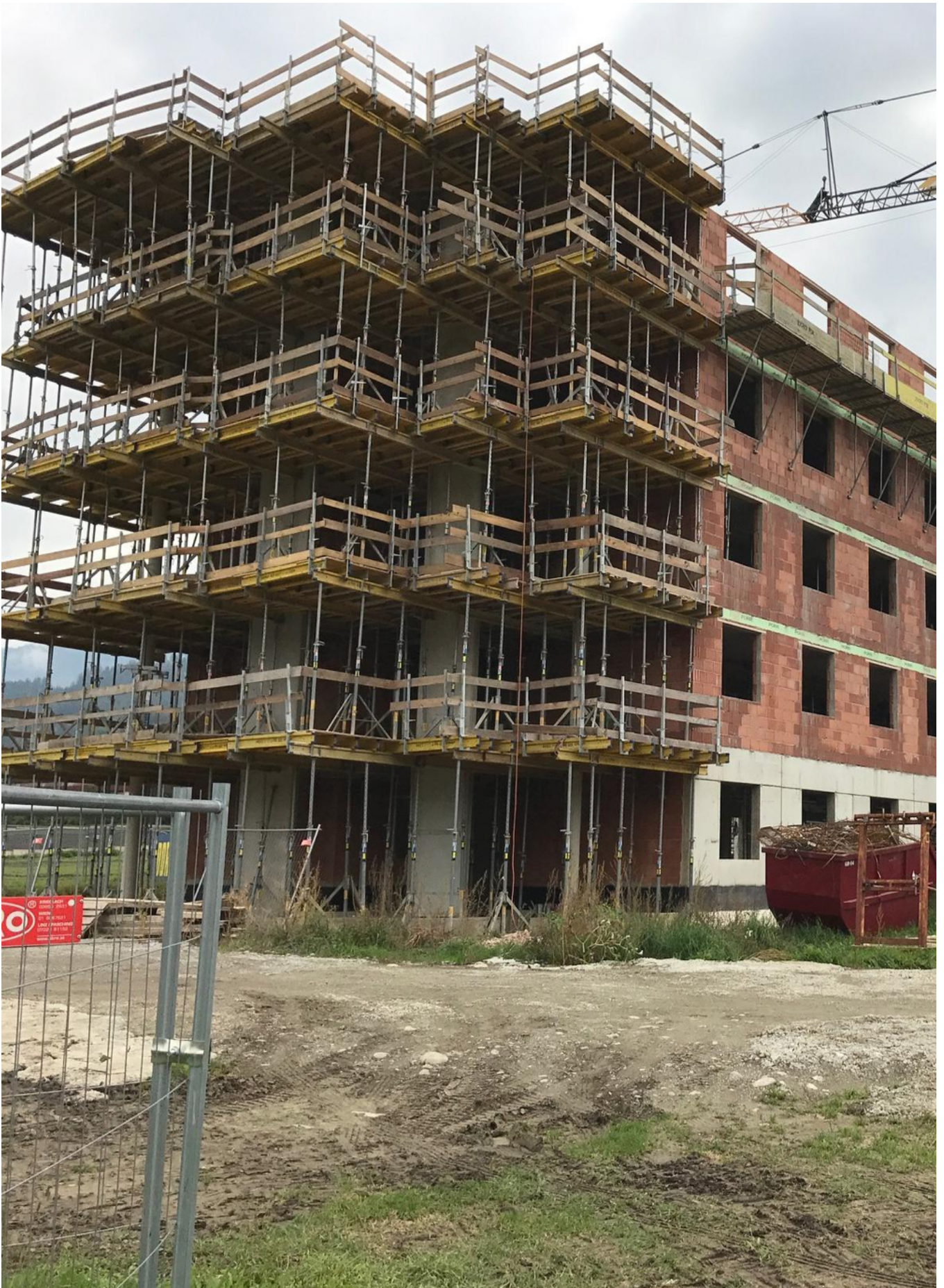
The external walls and the load-bearing walls in the vicinity of the staircases are composed of vertical coring bricks. Source: PORR
