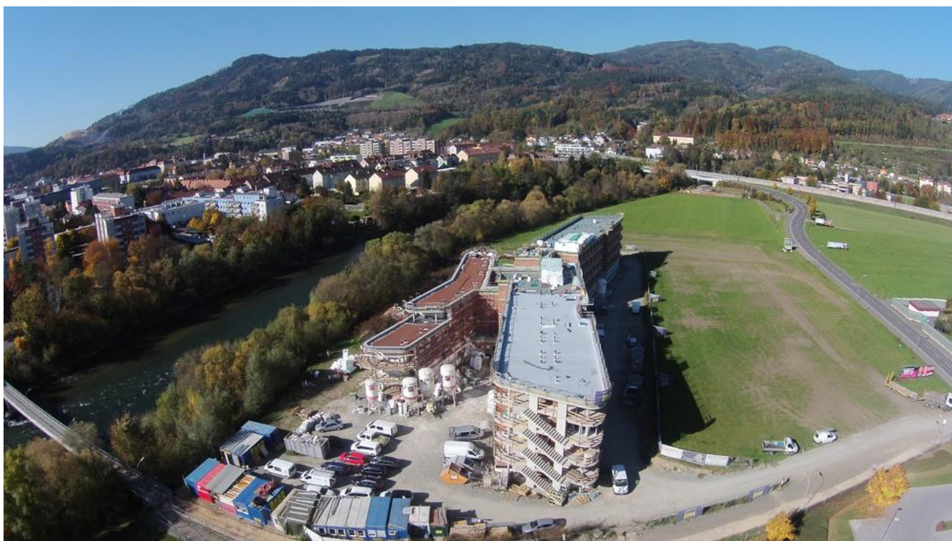
The building features flat roofs in all areas. The shorter of the two main building sections features an extensive green roof. Source: PORR
