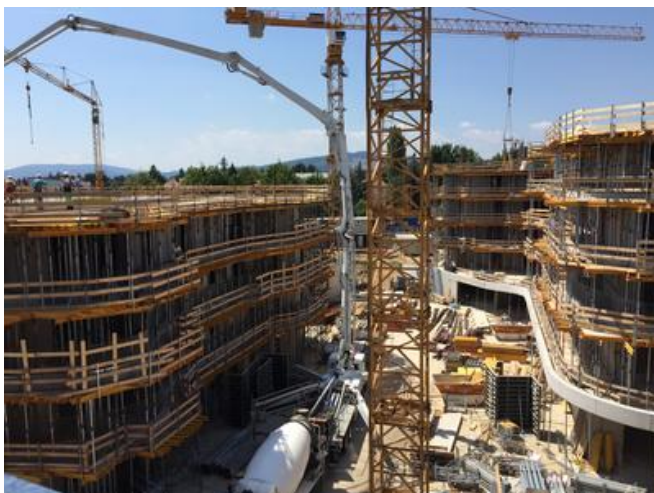
The formwork for the 3 km of balcony edge beams presented a particular challenge. Source: PORR
