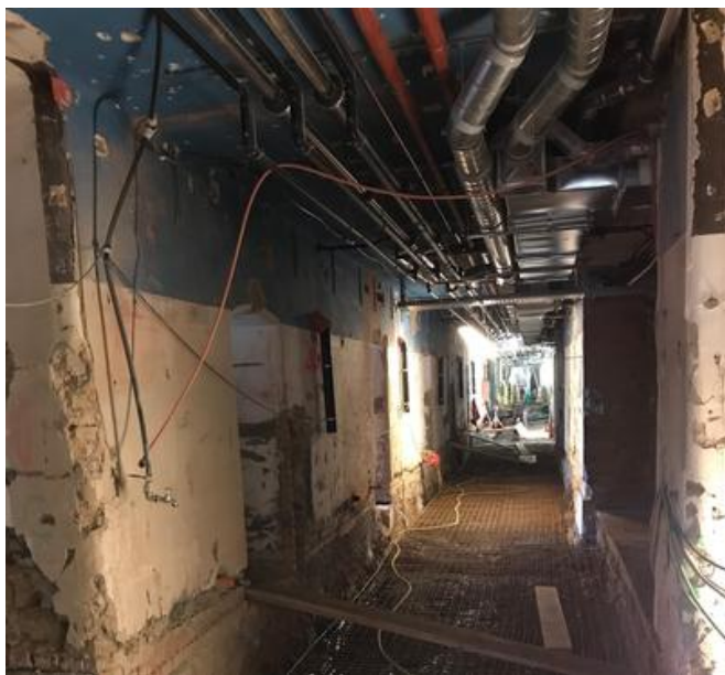
The metre-thick brick walls in the lower floor were dried out using injections. Source: PORR
