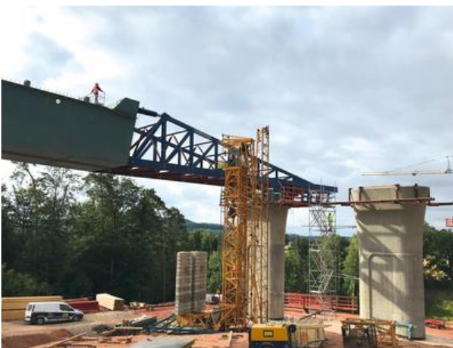
Components including the launch rockers, a launching nose for shifting the individual sections and a launch system including a lateral slide strand jack of our own design were developed from scratch and can now be used for other projects. Source: PORR
