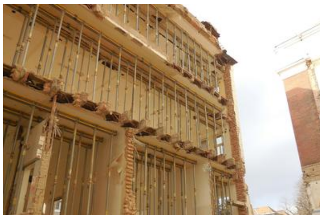
The ceilings had to be shored up and secured with underpinnings several times during the demolition work. Source: PORR
