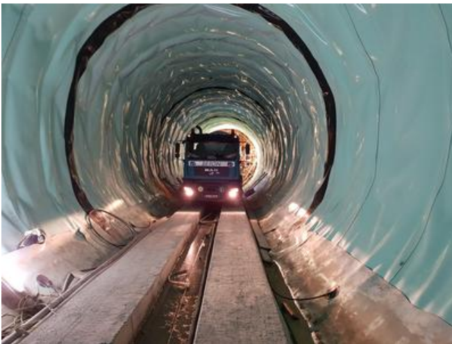
The sealing work was carried out in parallel with the concrete production, during night shifts. Source: GKI PRB consortium
