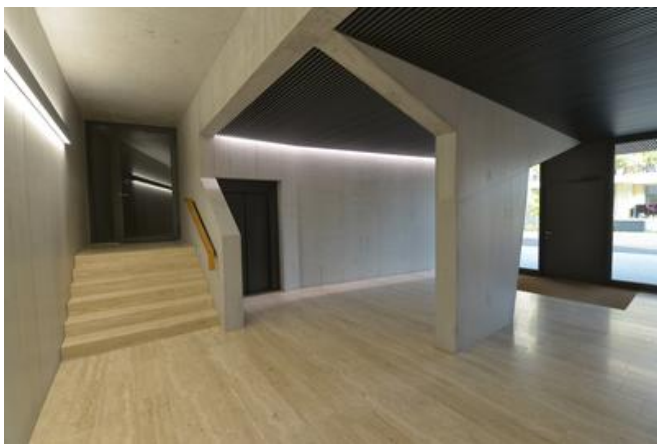
The finished entrance hall with its striking concrete column: an invisible connection to the ceiling was facilitated using a reverse bending connection. Source: PORR
