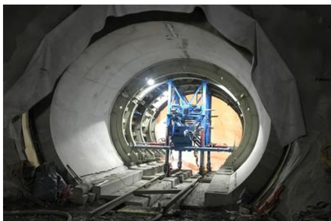
The tunnel invert and roof were concreted after installation of the membrane seal. Source: PORR
