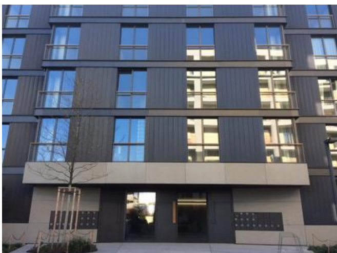
Instead of using a standard product, PORR manufactured all the metal facade sheets individually. Source: PORR
