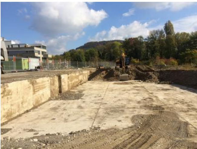
The dry construction pit with old building structures, which were retained. The new basement was built into the old structure and sealed to form the white tank system. Source: PORR
