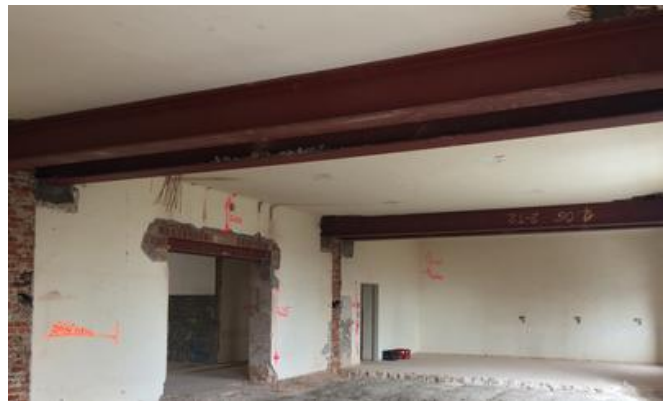
Internal supporting walls had to be removed from the large dining hall and the ceilings underpinned with steel beams. Source: PORR
