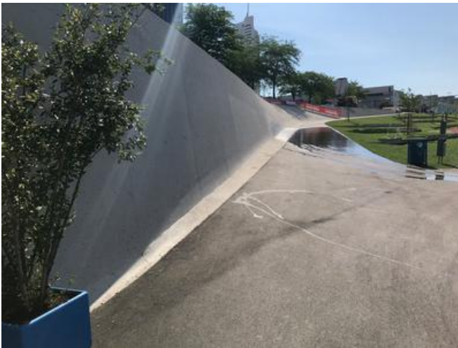
Custom-made formwork was needed to produce the exposed concrete surfaces. Source: PORR
