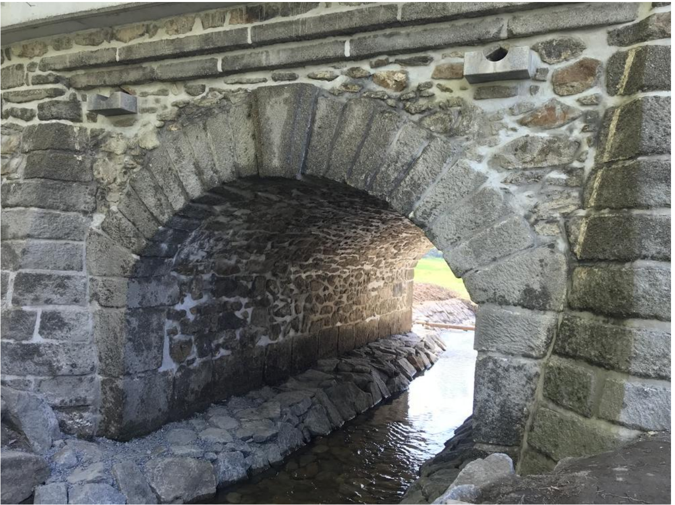
The visible areas of jointing were neither smoothed nor treated in any other way. Missing parts of the natural stone masonry were filled in using rubble. Source: PORR
