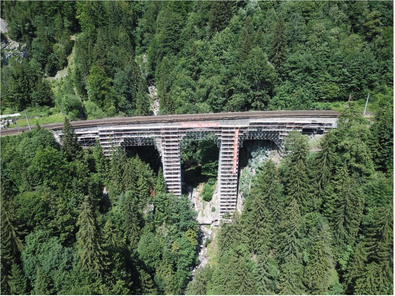
A total of 320t of material was used for scaffolding the Schmiedtobel viaduct. Source: PORR
