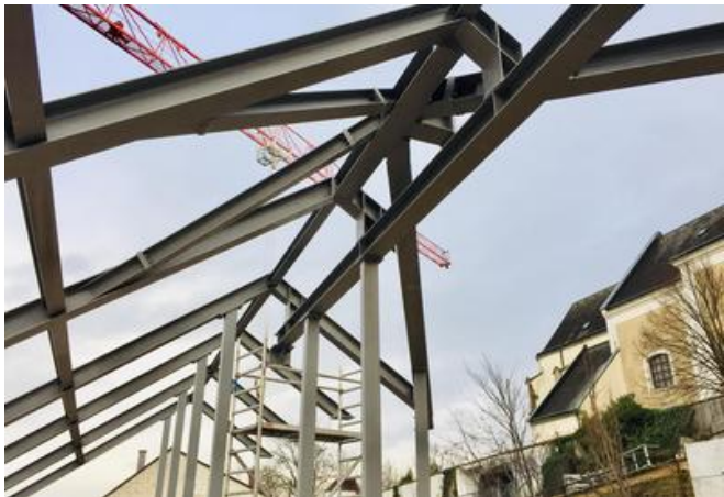
The new roof framework required a steel construction as the uppermost cornices of the old town hall featured a rooflight throughout. Source: PORR
