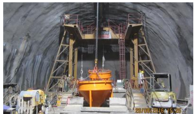
The working platform for the poured concrete was subsequently used as a platform for all the shaft work. Source: GKI PRB consortium
