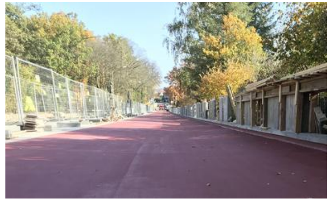
Caption: A new road surface was applied on the bridge and its ageing concrete rails were replaced. Source: PORR
