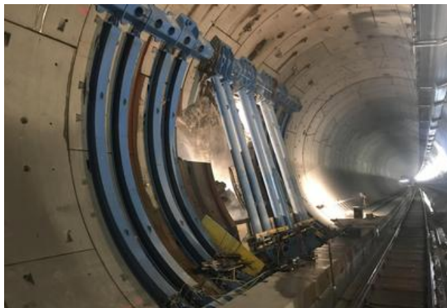
Before breaking through for the cross sections, the lining segments in the Neogene zone were shored up with steel reinforcement. Source: PORR AG
