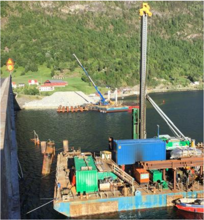
The piles being driven. In the background, 14 fully installed piles for another foundation can be seen. Source: PNC Norge AS
