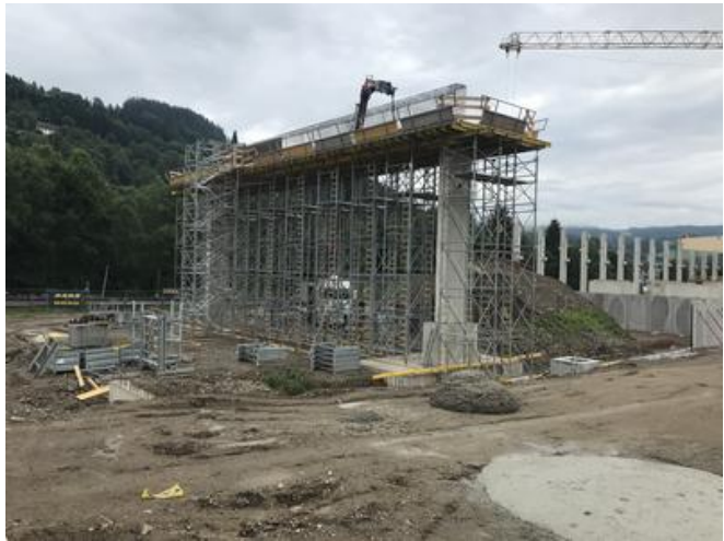
Due to their high dead load, the girders could not be delivered as pre-cast components, as specified in the tender, but had to be constructed in-situ instead. Source: PORR
