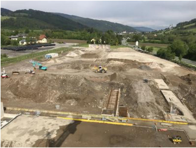
Up to five excavators and a wheel loader were in constant use during the earthworks. Source: PORR
