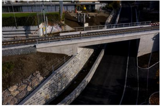
The completed bridge over the Mänibach Stream. Source: PORR
