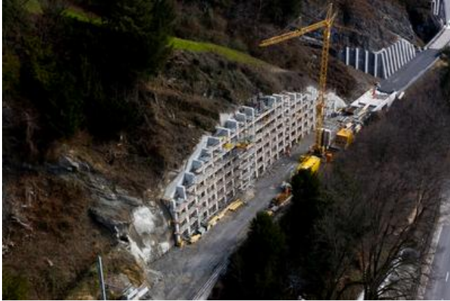
The team built extensive supporting structures in section 3. Source: PORR
