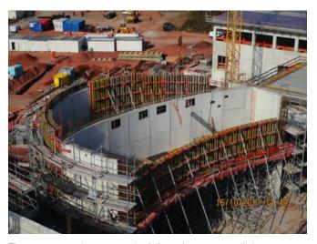
The stage tower has a curved reinforced concrete wall that was a significant challenge to build. Source: BBGS GmbH
