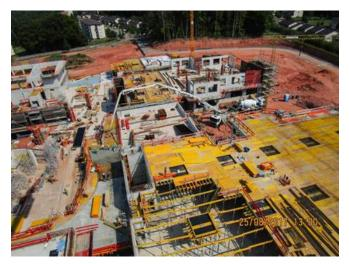
In order to meet the high security requirements, the school was built almost entirely using a monolithic construction technique. Source: BBGS GmbH
