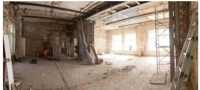
...and during the conversion work Source: PORR
