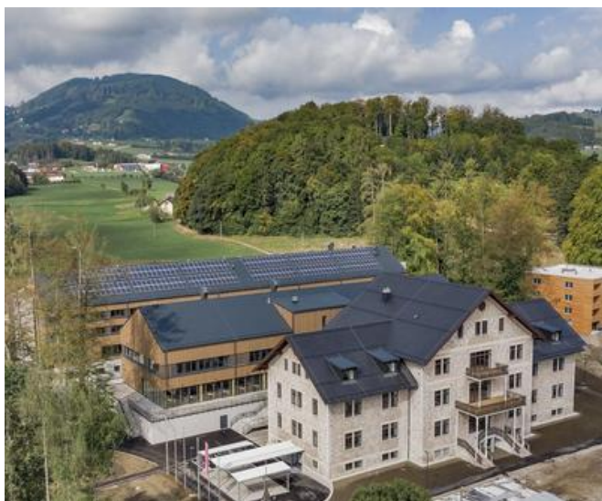
The original building is in the foreground; behind it can be seen the new timber buildings with solar panels on the roof. Source: Gerd Kressl
