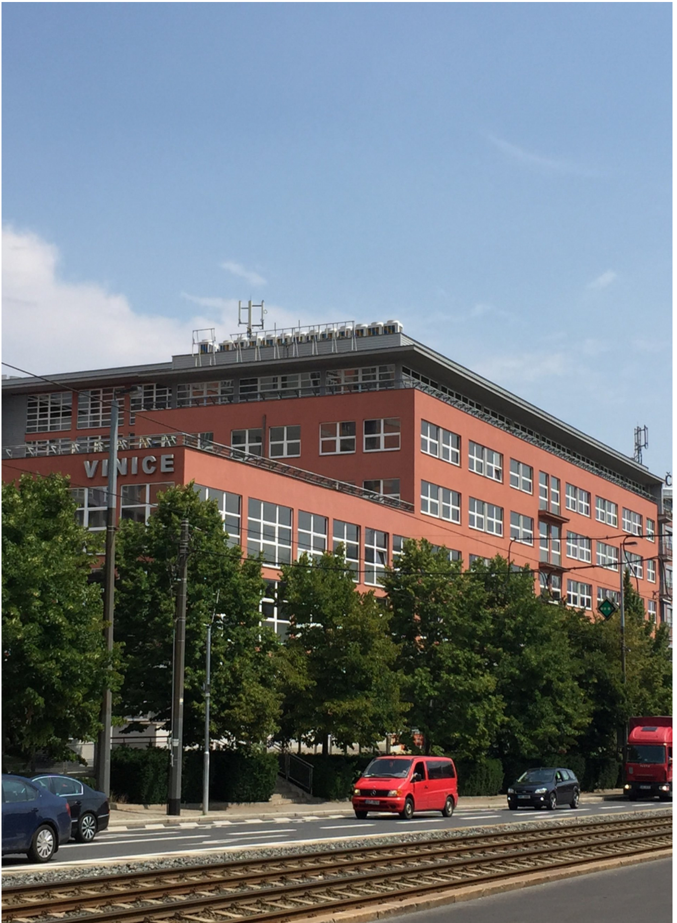
PORR is transforming an old 90s office building into the new home of one of the Czech Republic's leading media companies. Source: PORR
