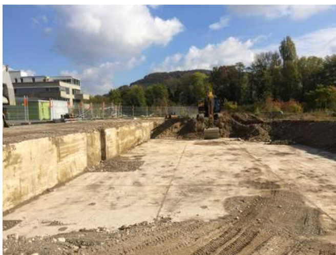
The dry construction pit with old building structures, which were retained. The new basement was built into the old structure and sealed to form the white tank system. Source: PORR
