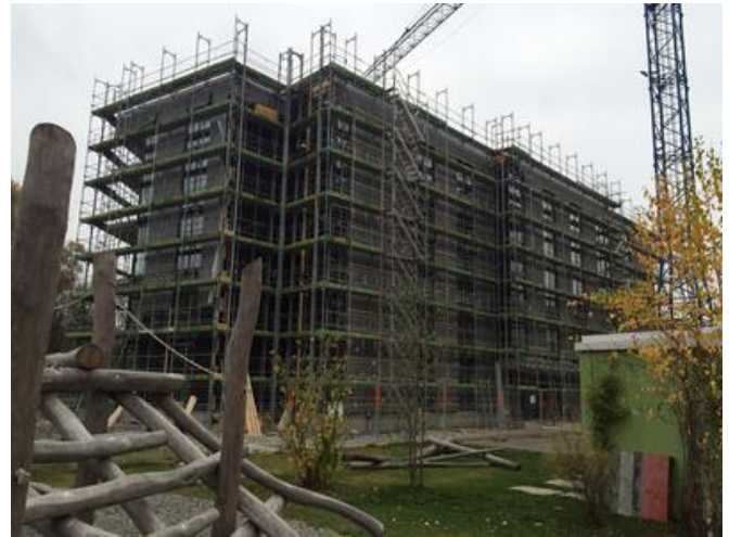
The carcass prior to installation of the ventilated facade. Source: PORR
