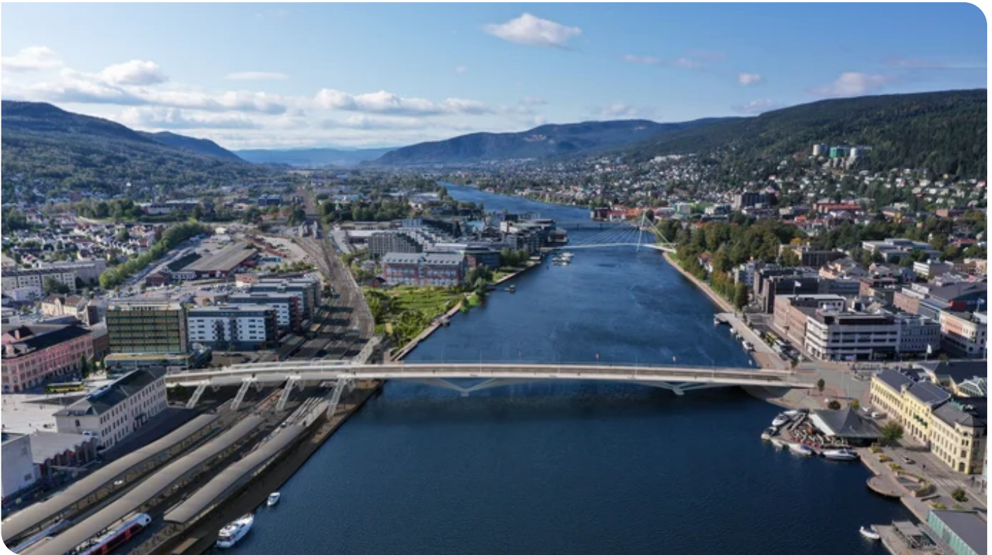
During the construction of the Bybrua in Drammen, Norway, the passing salmon must not be disturbed. (c) PORR
