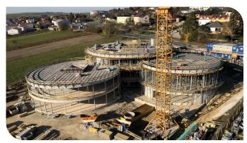
The floor plans of the three buildings are formed by intersecting circles. Spacious atriums are located at the respective centres of the circles. (c) PORR
