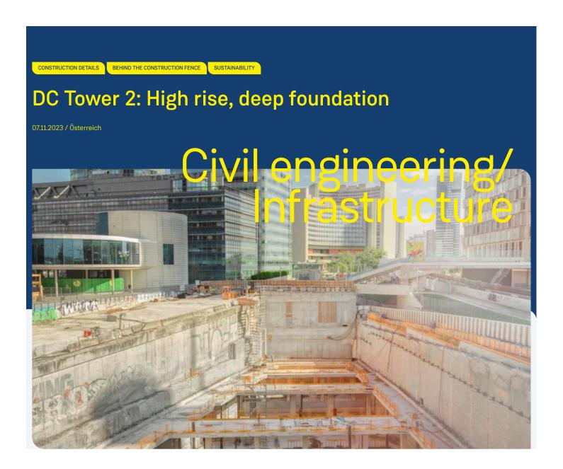
PORR's special civil engineering team dug 22.7 metres into the ground for DC Tower 2 in Vienna. This created a secure foundation for the tower.
