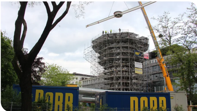
Lifting the 28m-long platform with central ring construction. (c) PORR
