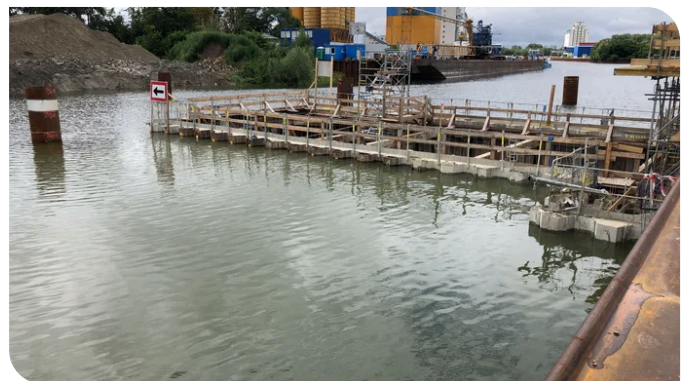
The sheet piling enclosures during construction phase, under flood conditions. (c) PORR
