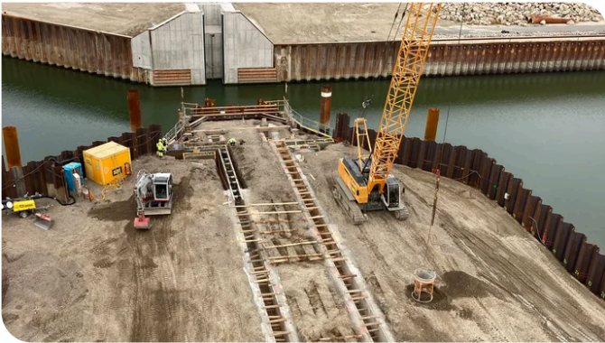
Preparations for work on the diaphragm wall in construction phase 2. (c) PORR
