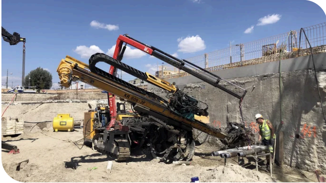
The diaphragm wall was anchored with 183 temporary anchors. Source: PORR
