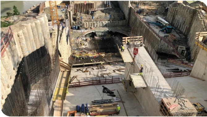
The base slab is nearly complete. Source: Thomas Wieczorek
