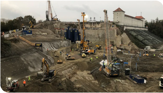
There were five pressurised aquifers that the construction pit work needed to take into account, with the pressure increasing with each aquifer. Source: Markus Trinkl
