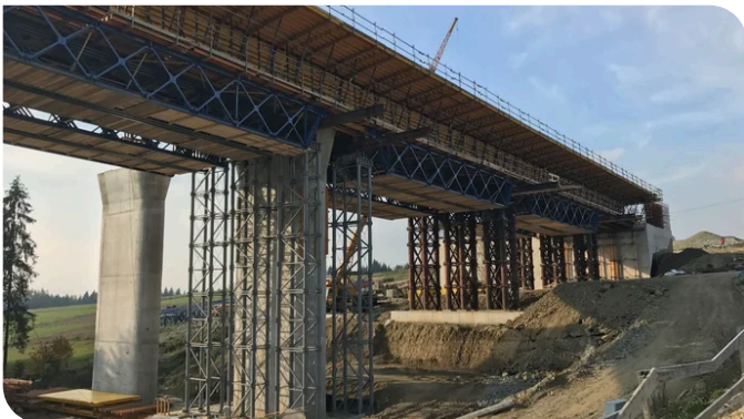
Load-bearing structure of the access part including support system. Source: PORR
