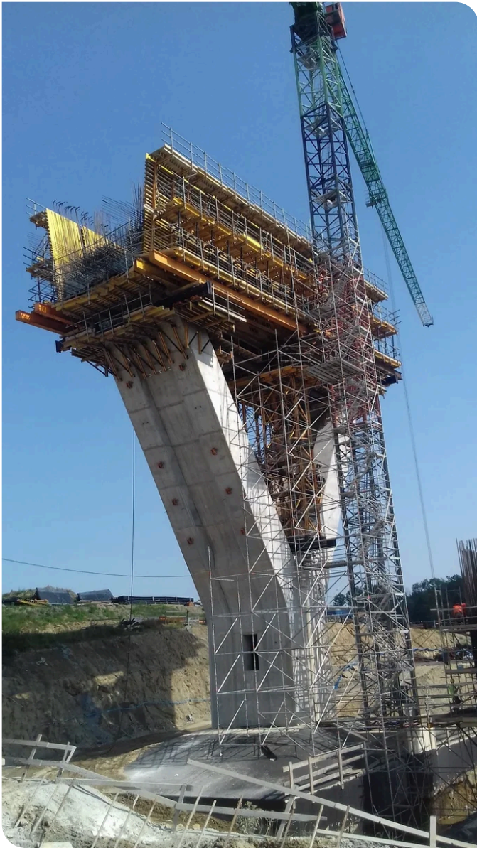
For construction purposes, the Y-shaped piers supporting the longest bridge spans were divided into the three sections: "pier shaft", "head" and "arms". Source: PORR
