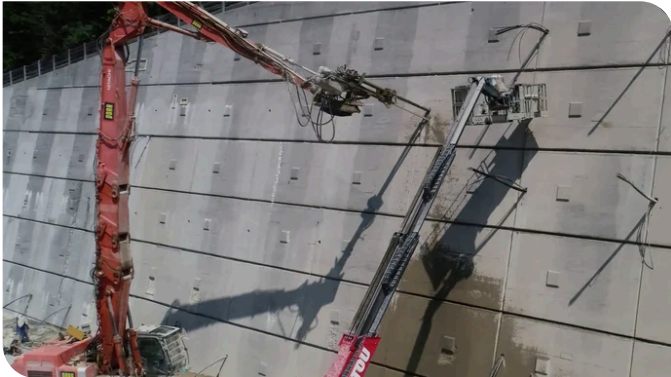
A 60t excavator with carriage attachment was used for drilling at heights of up to 20m. Source: PORR Specialist civil engineering
