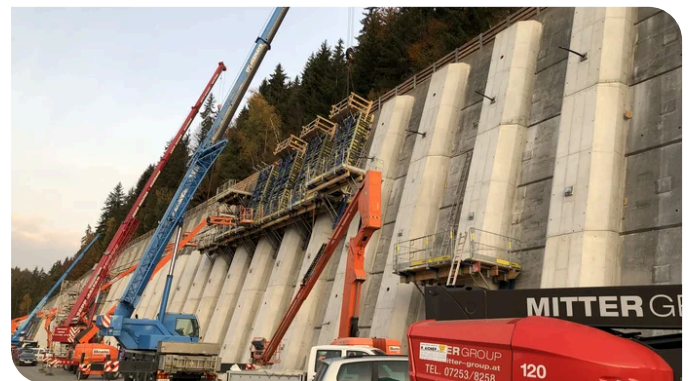
The pilaster strips on the anchor wall were concreted after the anchor holes had been drilled. Source: PORR Specialist civil engineering
