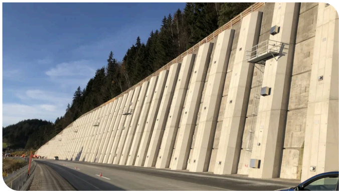
Regular monitoring of the anchor walls is facilitated by fifteen measurement cross-sections, fitted with 32 force plates and 25 extensometers. Source: PORR Specialist civil engineering
