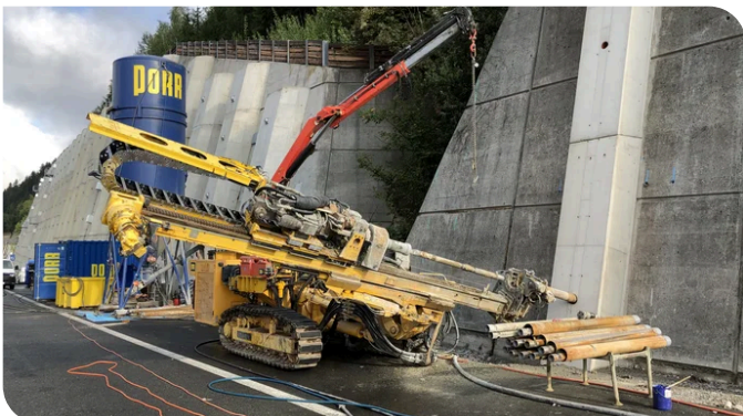
The drill holes in the lower level were drilled using a crawler drill rig. Source: PORR Specialist civil engineering
