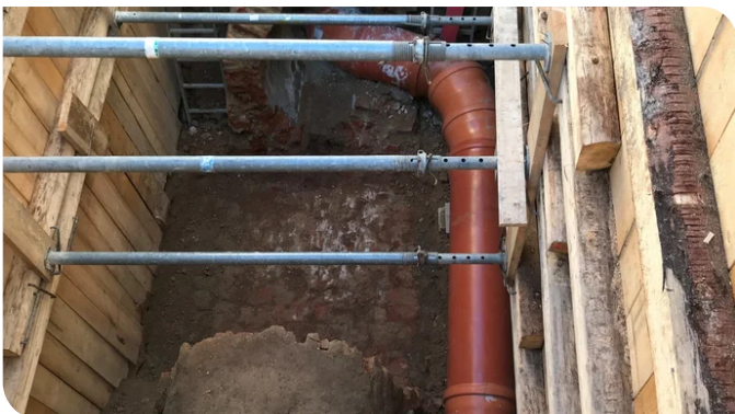
During the project, over 4,400m 3 of wooden trench shoring was installed. Eight new shafts were constructed as “white tank” constructions for the district heating. Source: PORR
