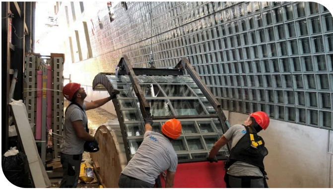
Hoisting the elements into place proved particularly challenging due to the cramped conditions. Source: PORR
