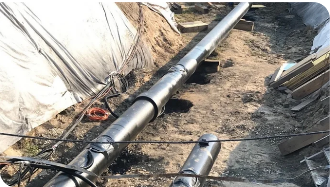
The damaged pipeline had to be excavated along a length of 140m in preparation for replacement. Source: PORR
