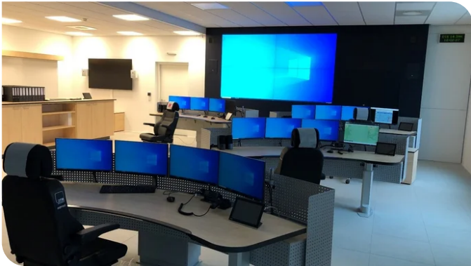
There is an earthquake-proof raised floor under the control room. Source: PORR
