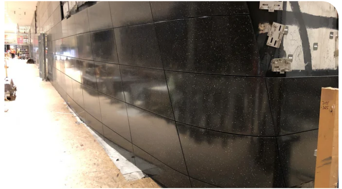
Every façade slab is slotted into its allocated place like a jigsaw piece. Source: PORR/Ilmert
