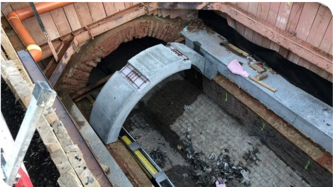
Positioning the precast concrete elements to close the brick vault of the Krottenbachkanal. Source: PORR
