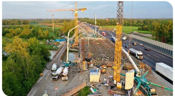
The delivery of concrete for concreting the superstructure proved to be a real challenge because of the high volume of traffic. Source: PORR
