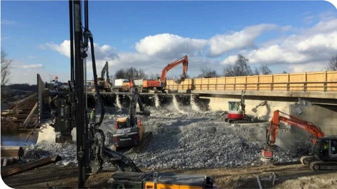
The existing superstructure is being demolished in the background, while the sheet piling work for the new construction is being carried out in the foreground. Source: PORR
