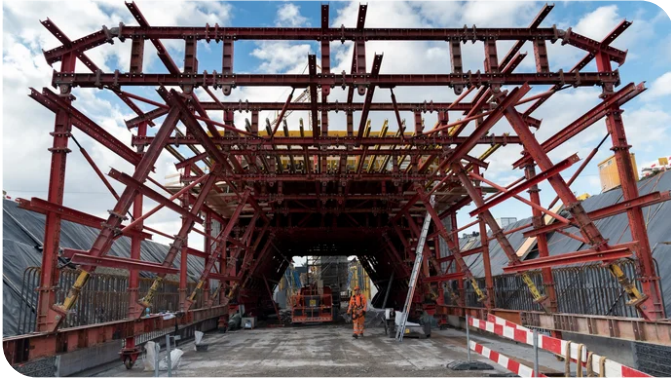
Formwork carriage and tracking carriage during assembly for the next 32 slab stages. Source: PORR
