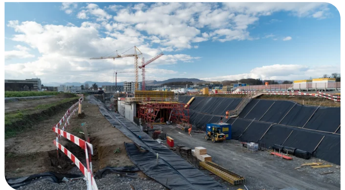
Start of the first stage of concreting the tunnel ceiling and tunnel entrance with formwork and curing carriages. Source: PORR
