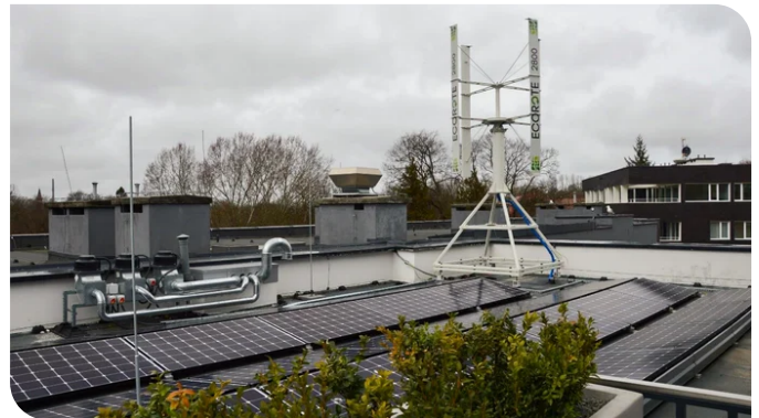
Several photovoltaic modules and a wind turbine on the roof provide clean electricity. Source: PORR
