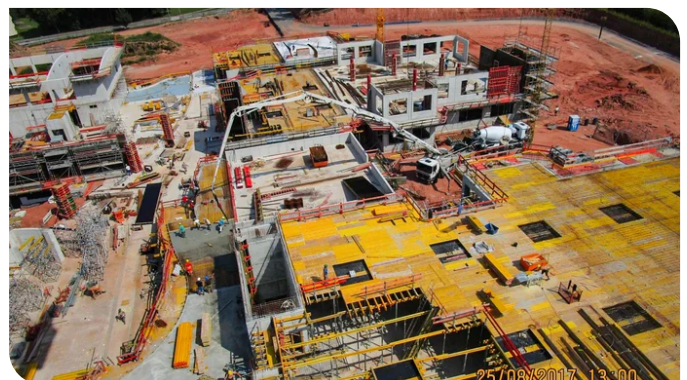
In order to meet the high security requirements, the school was built almost entirely using a monolithic construction technique. Source: BBGS GmbH
