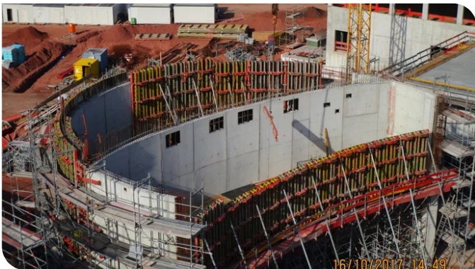
The stage tower has a curved reinforced concrete wall that was a significant challenge to build. Source: BBGS GmbH
