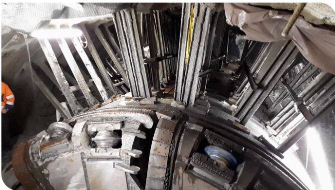
On several occasions, the trapped shield skin had to be released by raising the tunnel roof. Source: GKI Maria Stein consortium
