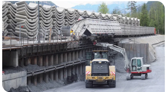
The GKI Maria Stein consortium took over the existing construction site from the previous contractor. Various restructures were necessary to improve efficiency – for example, the system for unloading spoil from the service carriages was completely reorganised. Source: GKI Maria Stein consortium
