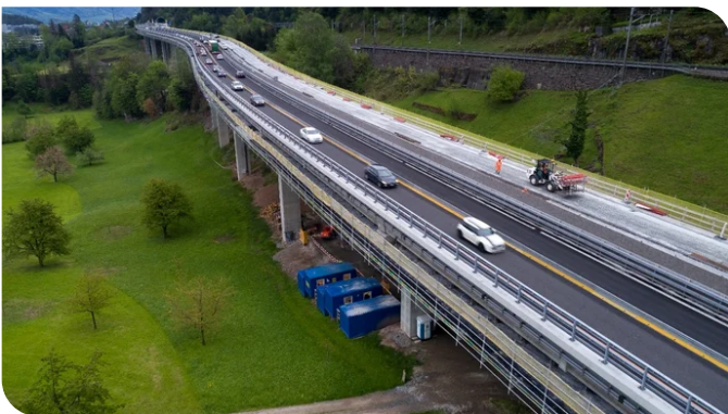
The Linden Bridge with scaffolding below the sides and new parapets. Source: PORR AG
