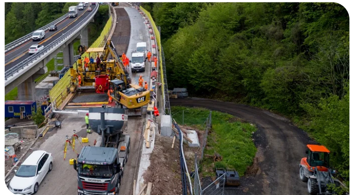
When temperatures during the day were high, work to apply the ultra-high performance concrete (UHPC) had to begin as early as 4am. Source: PORR AG
