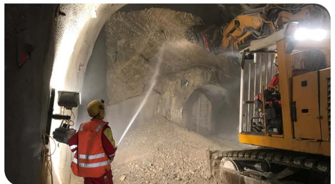
Work was carried out, using only an excavator, for the last few metres before reaching the west tunnel. Source: Thomas Exel
