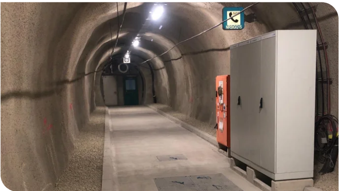
In addition to five vehicle-access cross passages, 15 pedestrian-access cross passages were also created. Source: Thomas Exel
