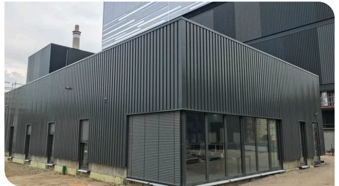
The entire power station will be monitored and controlled from the block control room building. Source: PORR/Fabian Hemauer
