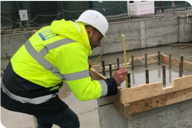
The rebars had to be placed with a maximum deviation of 5mm, in order that the grout sleeves could be assembled precisely on the prefabricated columns. Source: PORR Construct
