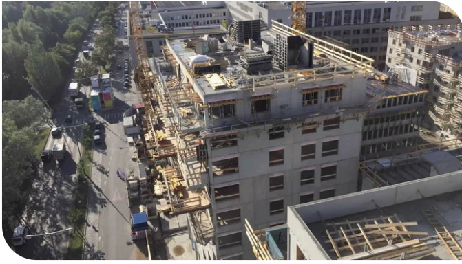
The overhanging balconies in the three top storeys presented a major challenge during the carcass construction. Source: PORR
