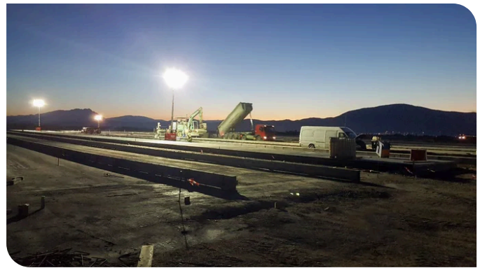
Solid steel girders were used as formwork for the concrete layer. Source: PORR Construct
