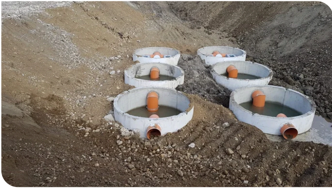
Water is cleaned in the two-stage oil separator system. Source: PORR Construct
