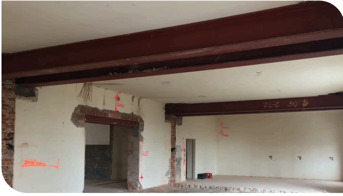
Internal supporting walls had to be removed from the large dining hall and the ceilings underpinned with steel beams. Source: PORR
