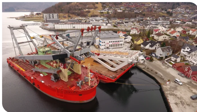
The first barge transported two bridge sections to the local quay near the construction site. The 800 tonne floating crane was also already on site at this time. Source: PNC Norge AS
