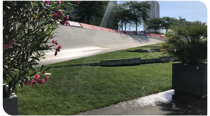
The straight retaining walls made of precast concrete elements invite people to linger with seating. Source: PORR
