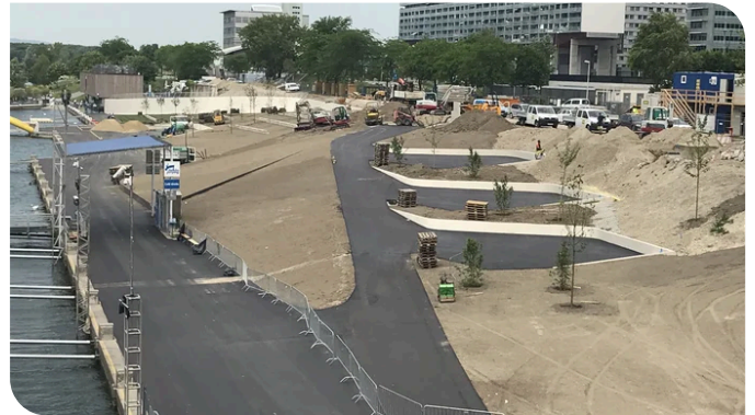
PORR erected several retaining walls featuring irregular curves along the embankment area. The largest retaining wall begins at the quay and ends at the top of the embankment (visible in the background). Source: PORR
