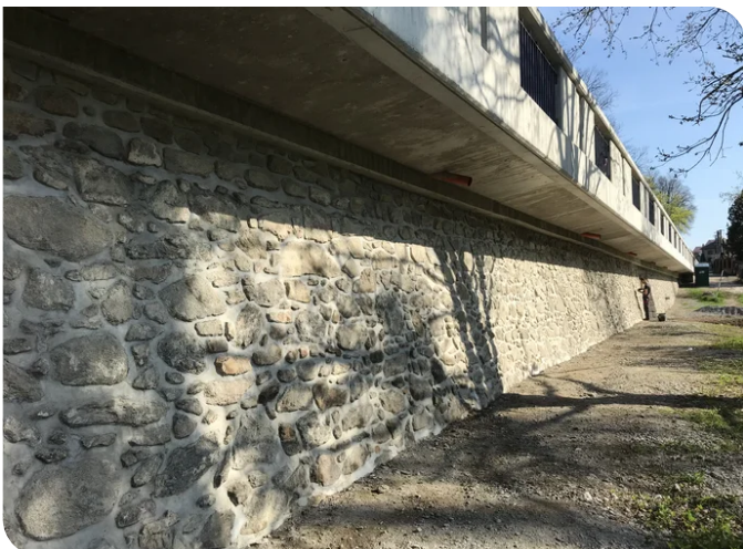
The bridge's foundations are made of natural stone. Source: PORR
