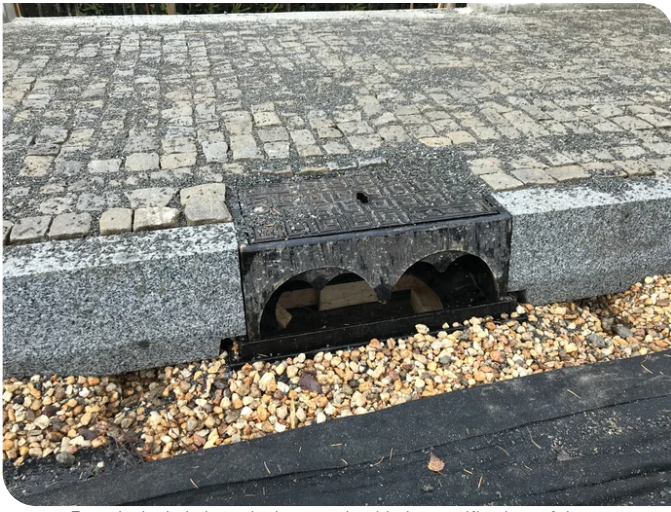
Even the kerb drainage had to comply with the specifications of the monument protection authority. Source: PORR
