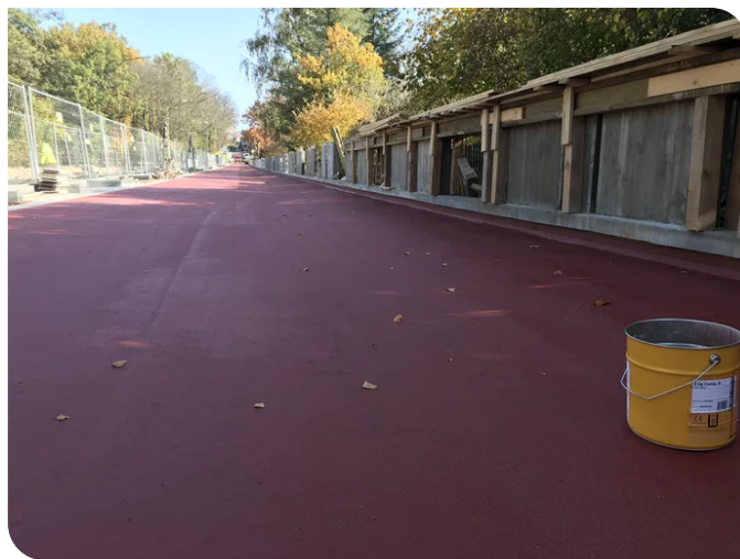
The bridge deck was replaced, as were the historic concrete railings. Source: PORR
