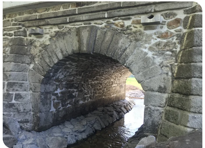
The visible joint surfaces were neither smoothed nor treated in any other way. Missing natural stone masonry was supplemented with quarry stone. Source: PORR
