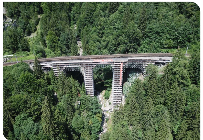
The Schmiedtobel viaduct was scaffolded with a total of 320 tonnes of scaffolding material. Source: PORR
