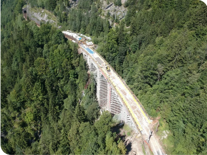
The entire structural renovation had to be carried out within a two-week track closure in August. Source: PORR
