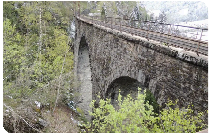
The Schmiedtobel Viaduct before the start of construction Source: PORR
