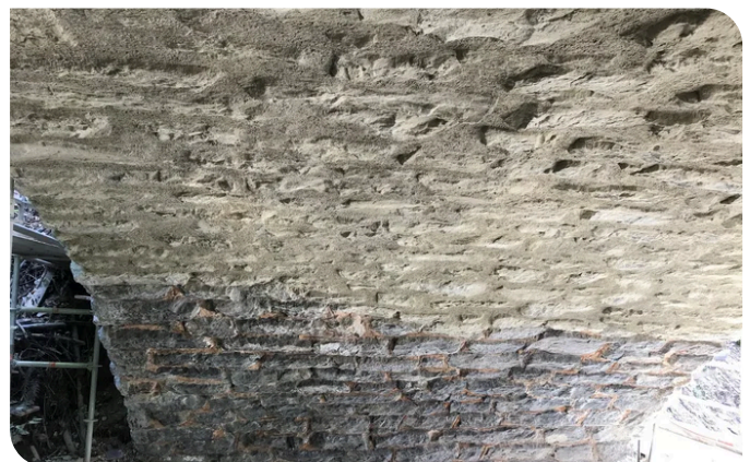
The entire masonry was cleaned with high-pressure water jets and then sandblasted. Source: PORR
