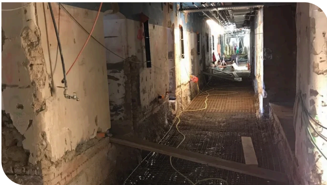
The metre-thick brick walls in the lower floor were dried out using injections. Source: PORR
