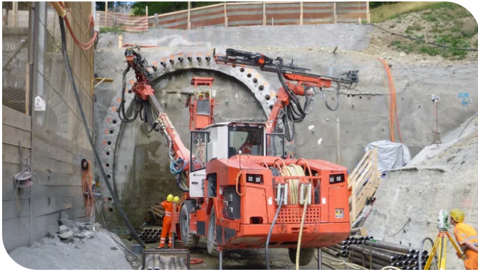
The railway line in Spinass continued operating during the pipe screen advance. Source: PORR
