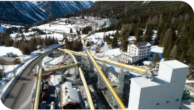
The consortium operates a gravel plant in Preda, which can process up to 4,000t of excavated material each week. Source: Torsten Schaarschmidt, Pöyry Schweiz AG
