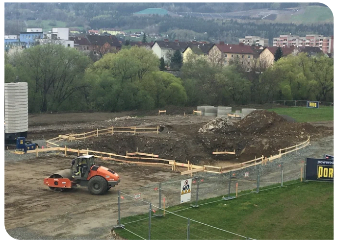
Dynamic pulse compaction was carried out to improve the soil conditions. Source: PORR
