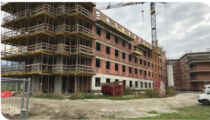
The exterior walls as well as the load-bearing walls in the stairwells are made of vertically perforated bricks. Source: PORR
