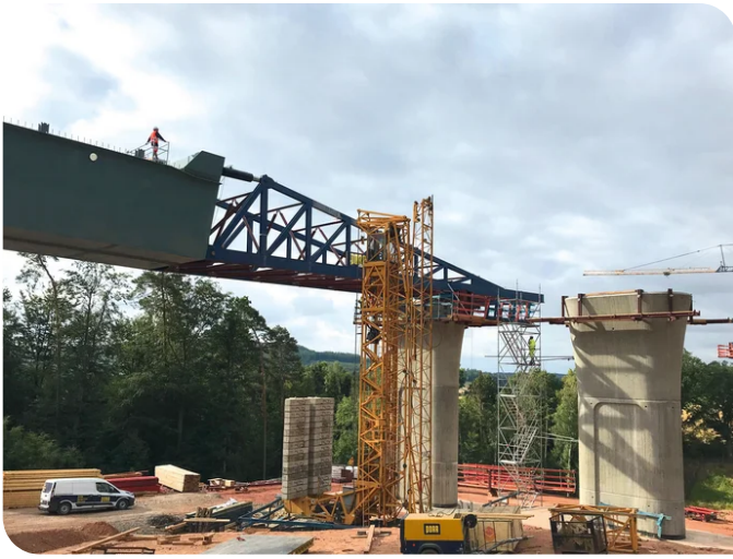
Components such as shifting rockers, a pre-construction beak for pushing the individual sections (image) or a pulling system with self-designed, horizontally operating strand jacks were newly developed and can now also be used for other projects. Source: PORR
