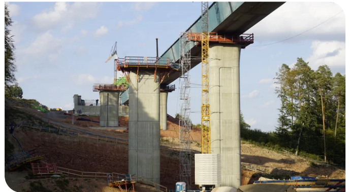
The piers have a height of almost 30 metres. Image source: PORR
