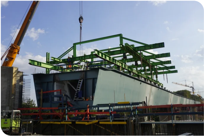
Erection of the formwork carriage (Weise Dortmund) for the production of the composite carriageway slab. Source: PORR
