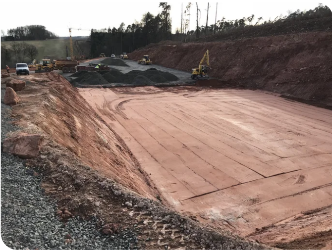
An excavation of around 25,000 cubic metres had to be removed for the cycle cellar and stored to the side for refilling. Source: PORR
