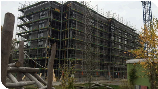
The carcass prior to installation of the ventilated facade. Source: PORR
