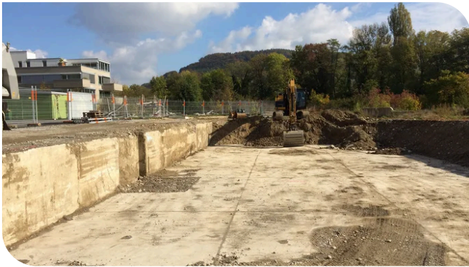
The dry construction pit with old building structures, which were retained. The new basement was built into the old structure and sealed to form the white tank system. Source: PORR
