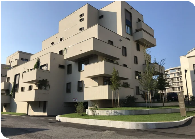
The completed Der Rosenhügel project was handed over to the client in May 2018. Source: PORR
