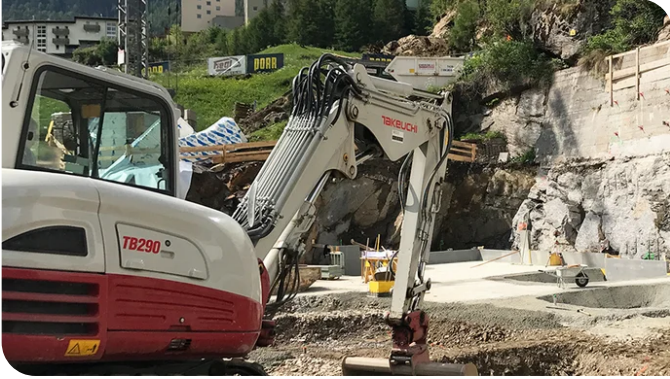
The construction pit was secured with jetcrete. Image: PORR AG
