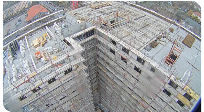
The supporting structure of the student residence was built using the bulkhead construction method. Image: PORR AG
