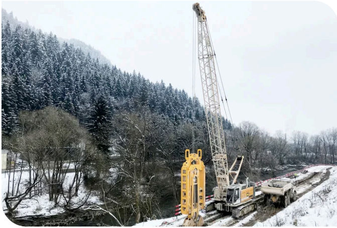
Installing the diaphragm wall. Image: PORR Bau GmbH
