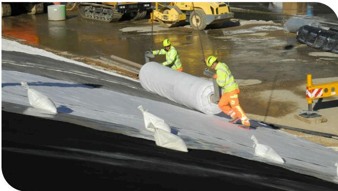
Laying the surface seal. Image: IAT GmbH
