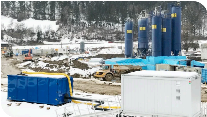
Soil gas extraction system (blue container) with a temporary exhaust line during ongoing site work. Image: PORR Umwelttechnik GmbH
