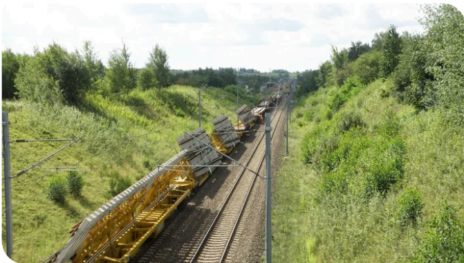
Transporting the switch blocks. Image: PORR AG
