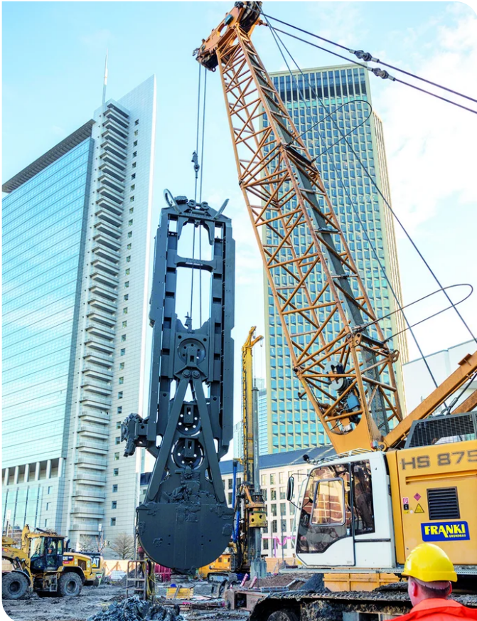
A diaphragm wall grab against a backdrop of Frankfurt's high-rise buildings. Image: FRANKI
