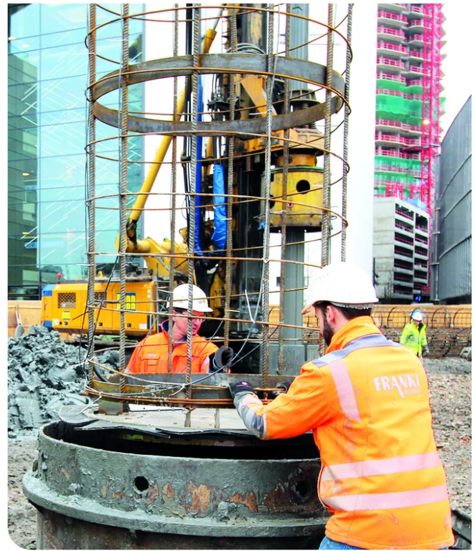
Pressure measuring pad for the foot before installation on the reinforcement cage. Image: isg
